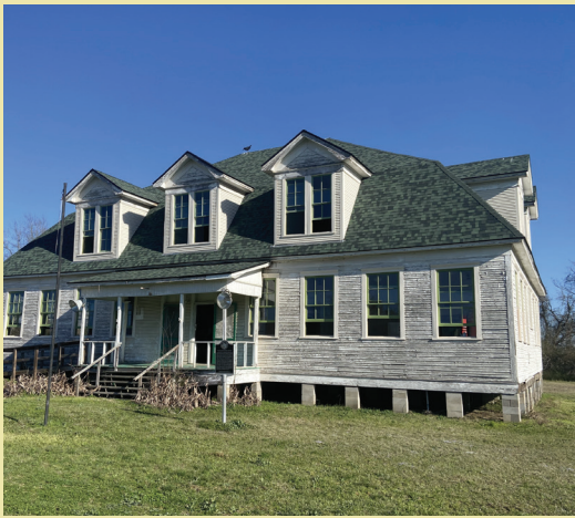
Wheelock School House - Before
